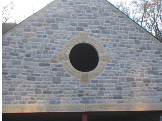
Fine sandstone masoned bullring window and keystone garage heads, to complement limestone walling
